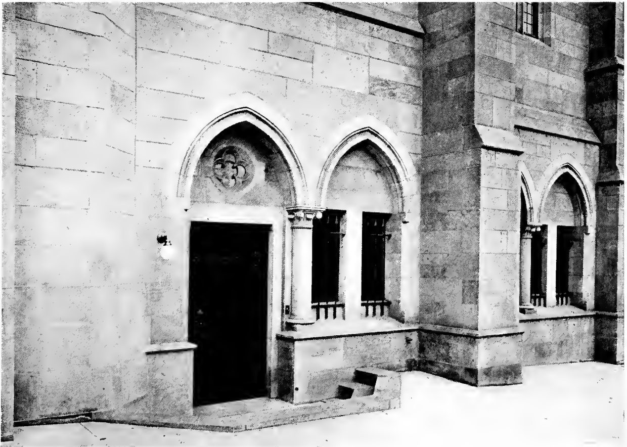
SYNOD HOUSE, CATHEDRAL OF ST. JOHN THE DIVINE, NEW YORK MESSRS. CRAM, GOODHUE & FERGUSON (BOSTON OFFICE), ARCHITECTS
